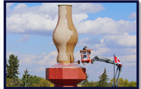
Donalda Gallery for the Arts & re-applying fiberglass on the Lamp Globe
